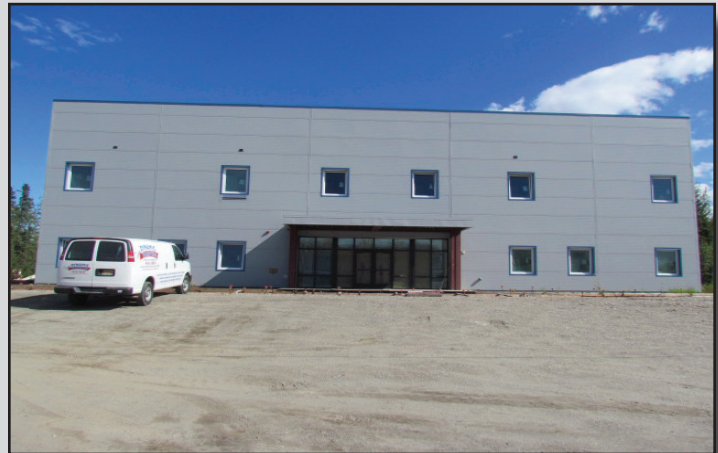
Fairbanks new training facility is finally complete!
